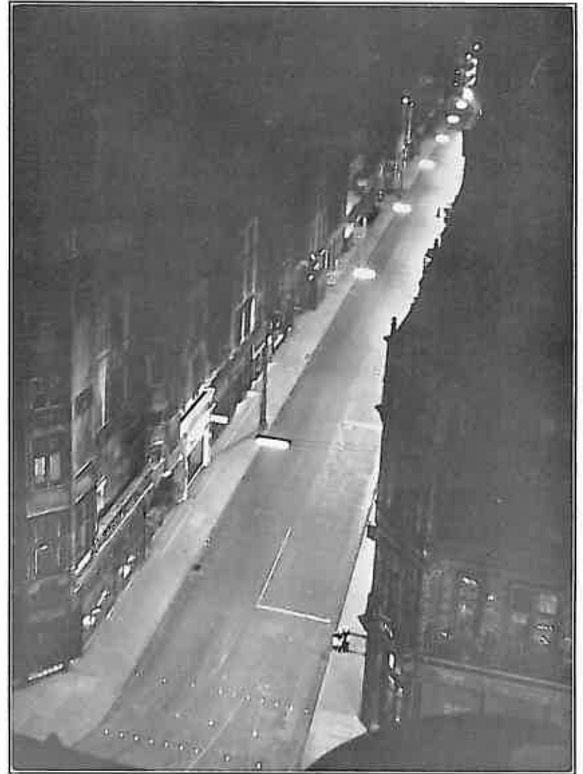
Fluorescent Street Lighting in Old Bond Street. Uses specially designed Mazdalux lanterns. This and High Street, Rugby, were the first tubular fluorescent lamp street lighting installations in this country, and the first of their kind in the world.
