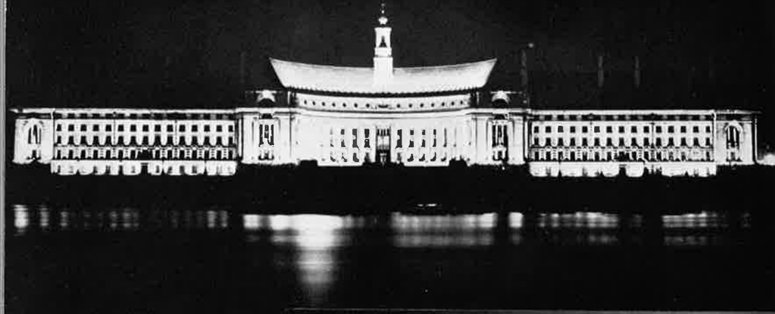
Left: COUNTY HALL, LONDON View from across the river showing floodlighting of London's administrative headquarters by means of Mercra Lamps in Mazdalux Floodlight Projectors.
