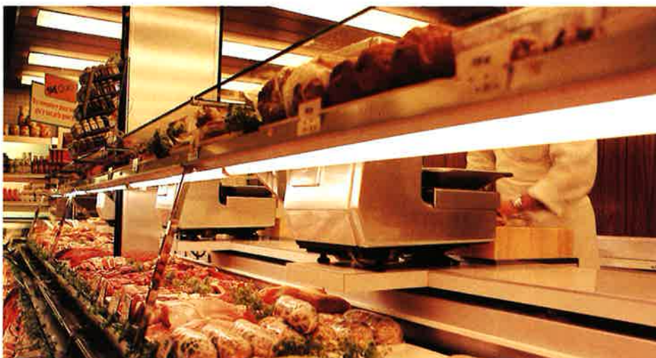
Natural fluorescent lamps enhance the red colours and are typically used in butchers' shops to display meat products to their full advantage.
